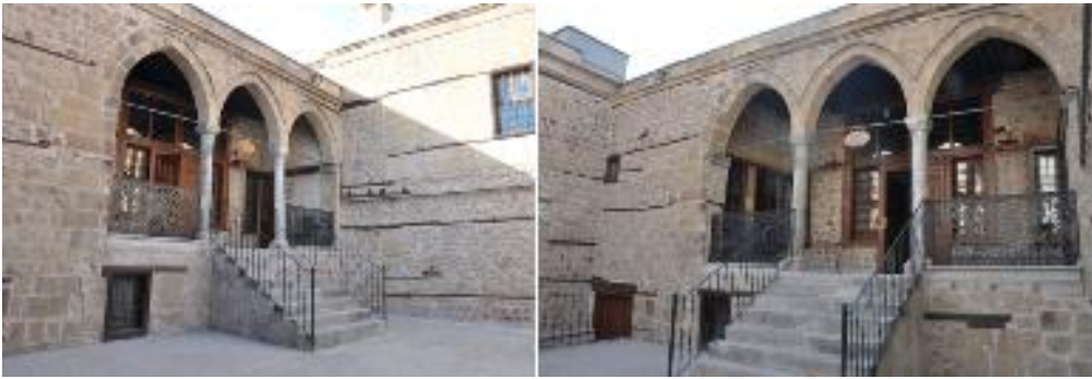
Figure 12. The courtyard of the traditional Niğde residence (Original, 2017)
