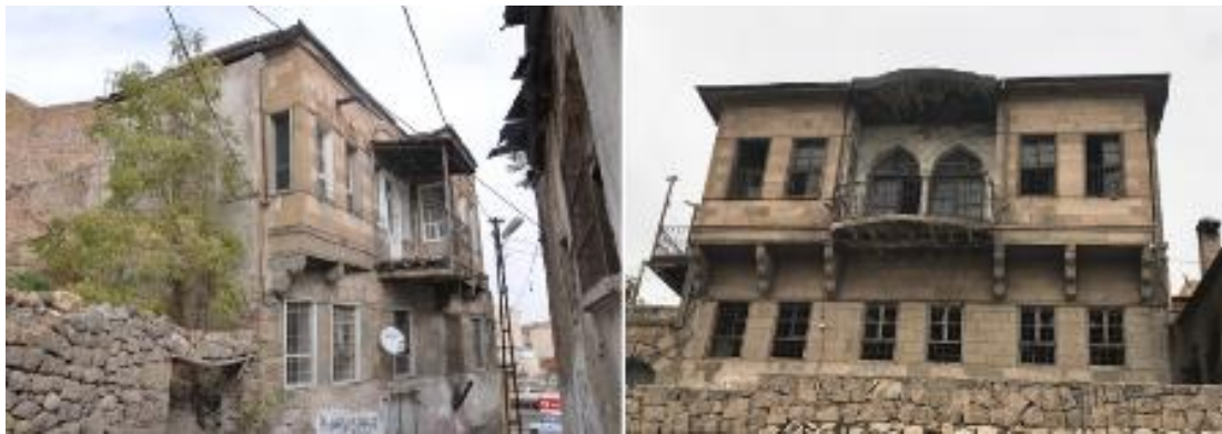
Figure 25. Neglected Residential Facades and Courtyard Walls (Original, 2017)
