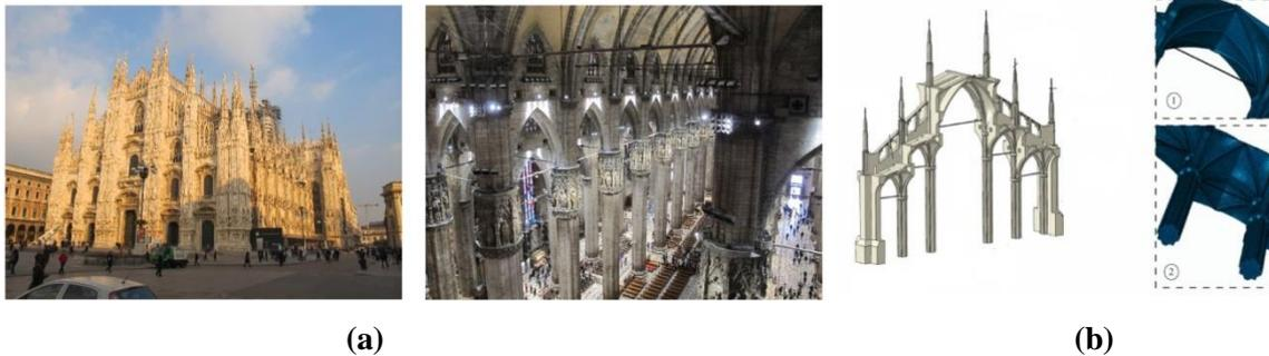
**Figure 5.** (a) External and internal view of Milan Cathedral, (b) Iron crossbars inside the church, **Source:** Angjeliu, Coronelli, Cardani and Boothby, 2020.
