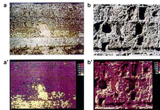
**Figure 18.** Determination of the structural character of the medieval city walls of Rhodes by digital image processing, **Source:** Moropoulou and others, 2013.
