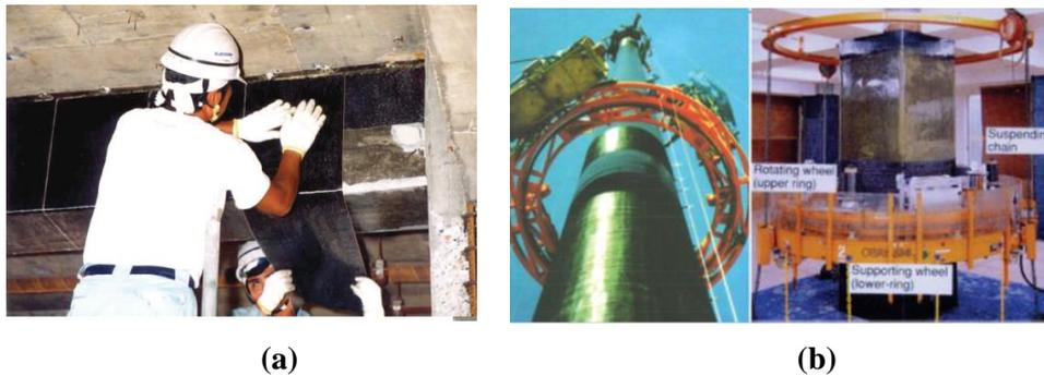
**Figure 2.** (a) Fibrous polymer application in beams, (b) Fibrous polymer application in columns, **Source:** Canbay, 2020.
