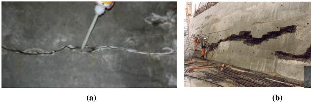
**Figure 3.** (a) Reinforcement application with epoxy resins, (b) Reinforcement application with repair mortar, **Source:** Canbay, 2020.
