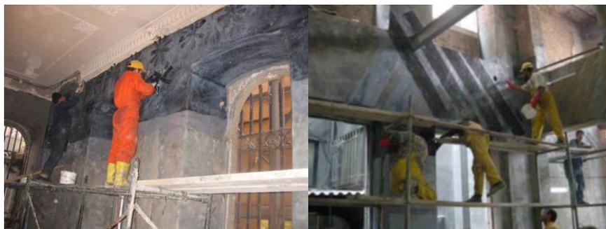
**Figure 7.** Reinforcement with fibre reinforced composites in historical buildings, **Source:** Peker, 2005.
