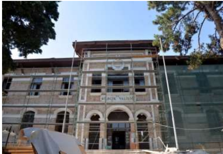
Photo 3. Governorate building restoration works (July 6, 2017) ( www.bilecik.csb.gov.tr )
