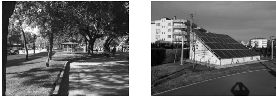
Figure 10. Application example of active (photovoltaic panel) and passive (solar control with trees) methods.
